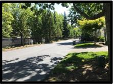
This line item is a provision to replace the asphalt seal coat on a 4-5 year cycle on the private roadway and parking area. This item however is for a 2nd coat on 9850 square feet of the total surface area. Life expectancy of overlay will vary depending how the Board of Directors strategize the maintenance for this line item including but not limited to seal coating at regular intervals.
