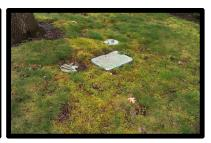
This line item is for the ongoing replacement of irrigation controllers and associated valves in the common area. Irrigation controllers should be replaced upon failure. Battery operated controllers typically have a life expectancy between 2-5 years. Electric operated controllers typically have a life expectancy between 5-8 years or longer. Component appears to be in fair condition, however should be tested by the contracted landscape company for an accurate assessment.
