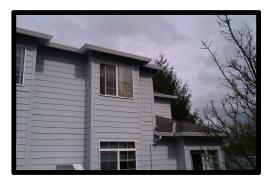
This line item is for the painting of the exterior siding. Existing paint appears to be in good to fair condition based on a visual observation. Information provided by the Board indicates that the siding was last painted in September 2014.
