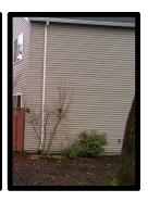
This line item is for the gutters and downspouts including elbows and fastening components for all condominium buildings. Replacement should ideally coincide with the roof replacement. Cost is per recent pricing information from Citywide Gutters in Portland, Oregon for similar components. (not a site specific bid) Gutters appear to be in good to fair condition based on a street-level visual vantage point.
