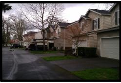
This line item is for the possible replacement of the fiber cement siding on 8 select buildings including some garages. The siding appears to be in fair condition based on a ground-level visual observation.
