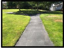
This line item is for the renewal of the asphalt walking paths. This includes the application of a bituminous overlay which normally is applied in one and a half inches to two inches thickness. This renewal of the overlay is designed to renew the life cycle of the pavement. The asphalt is in good condition in several areas and should be seal coated on a regular 4-5 year cycle to archive the maximum life expectancy.
