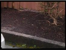
This line item is for replacement the concrete curbs and vehicle stops. Concrete has a life expectancy exceeding 30 years, however, there is some breakage that occurs over time due mainly to vehicles repeatedly slamming into these objects over time.
