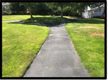
This line item is a provision to replace the asphalt seal coat on a 4-5 year cycle on the walking areas. Life expectancy of overlay will vary depending how the Board of Directors strategize the maintenance for this line item including but not limited to seal coating at regular intervals.
