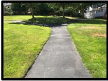
This line item is for the maintenance of the asphalt overlay in the walking areas of the community during each seal coat cycle. Overlay surface appeared in fair condition and should be seal coated every 3-5 years in order to maximize life expectancy
